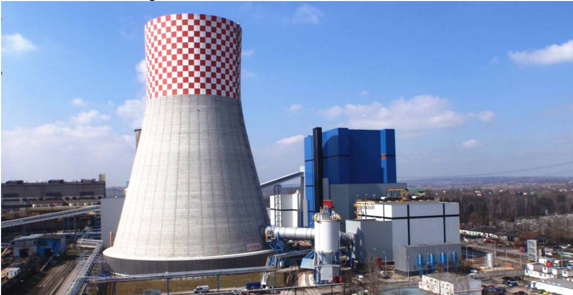
Figure 1-10: 460 MWe Łagisza super-critical CFB OTU Unit (FW report)
