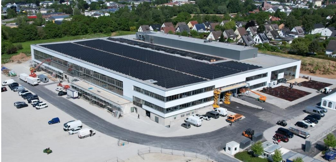
Figure 4 View of new Phoenix Contact technology and production building G60
