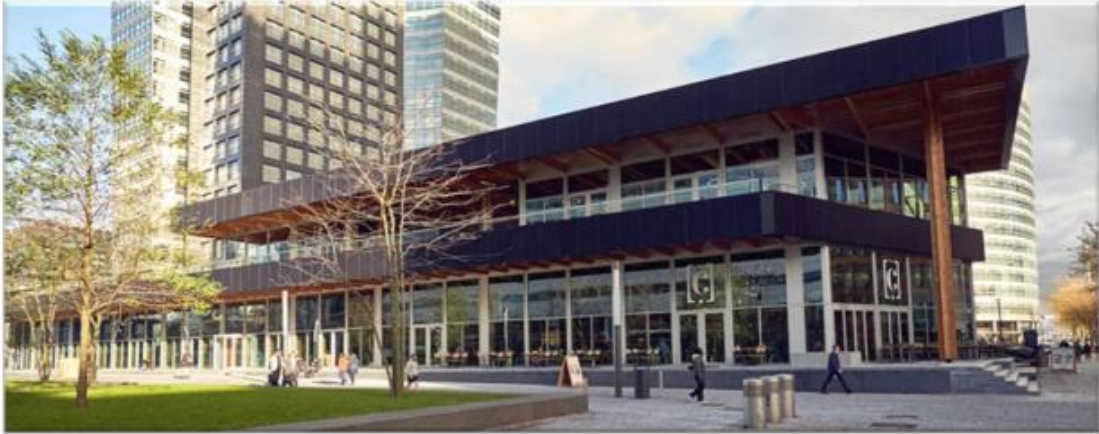
Figure 7 DC-powered Circl building in Amsterdam, The Netherlands
