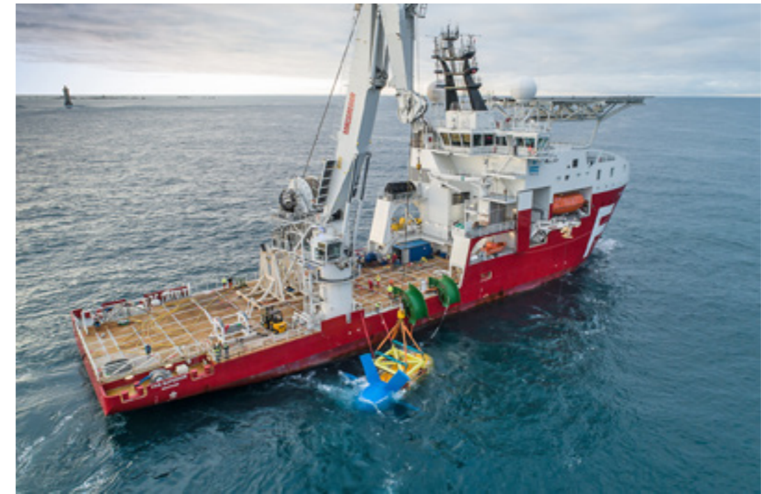
Figure 1: Deployment of D10-1000 turbine in the Fromveur Passage in October 2018. Source: SABELLA / Balao
