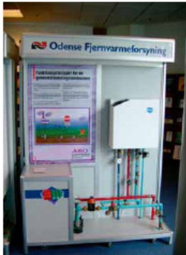
A typical consumer substation to a one-family house in the show room of the district heating company. The consumers are able to ask for advice before they decide to invest. The flow meter and valves in the left corner below belong to Odense District Heating Company, whereas the heat exchanger for hot tap water, the differential pressure valve, and other components belong to the consumer.
