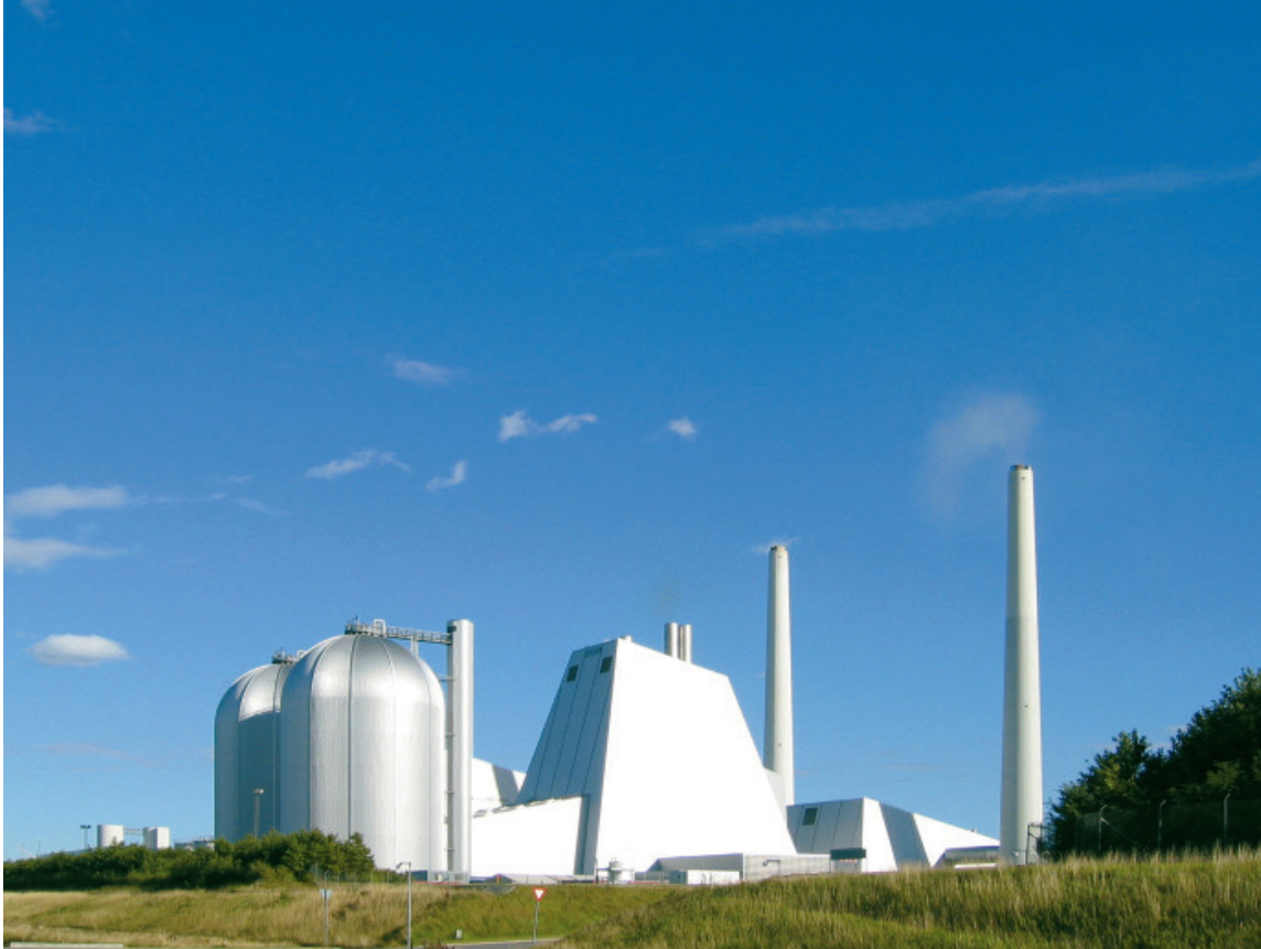
Figure 10-3 Heat accumulators at Avedøre Power Station situated at Avedøre Holme south of Copenhagen. The overall production capacity of the two Avedøre Power Station units is 810 MW of electricity and 915 MW of heat. 126
