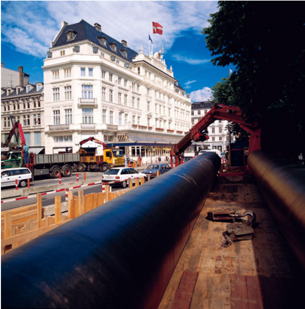
Figure 12-2 Installation of transmission pipelines in Central Copenhagen. 149
