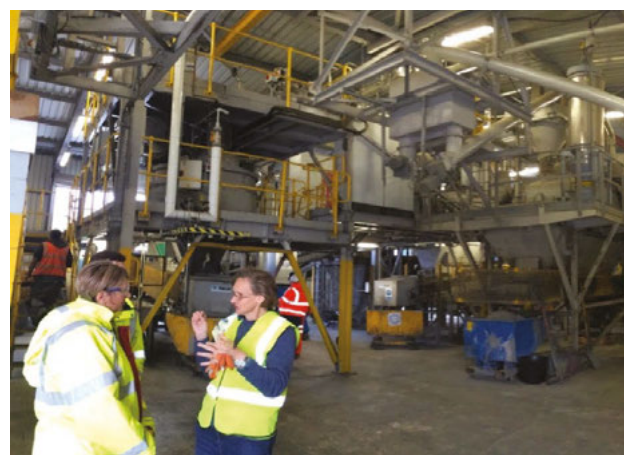
Figure 1: The Suffolk carbonated aggregates plant
