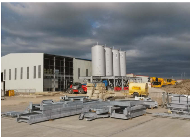
Figure 2: The C8 Avonmouth plant under construction, Summer 2015
