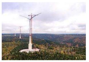
Figure 4 Gaildorf wind farm featuring four turbines with up to 178-m hub height. Source: Max Bögl
