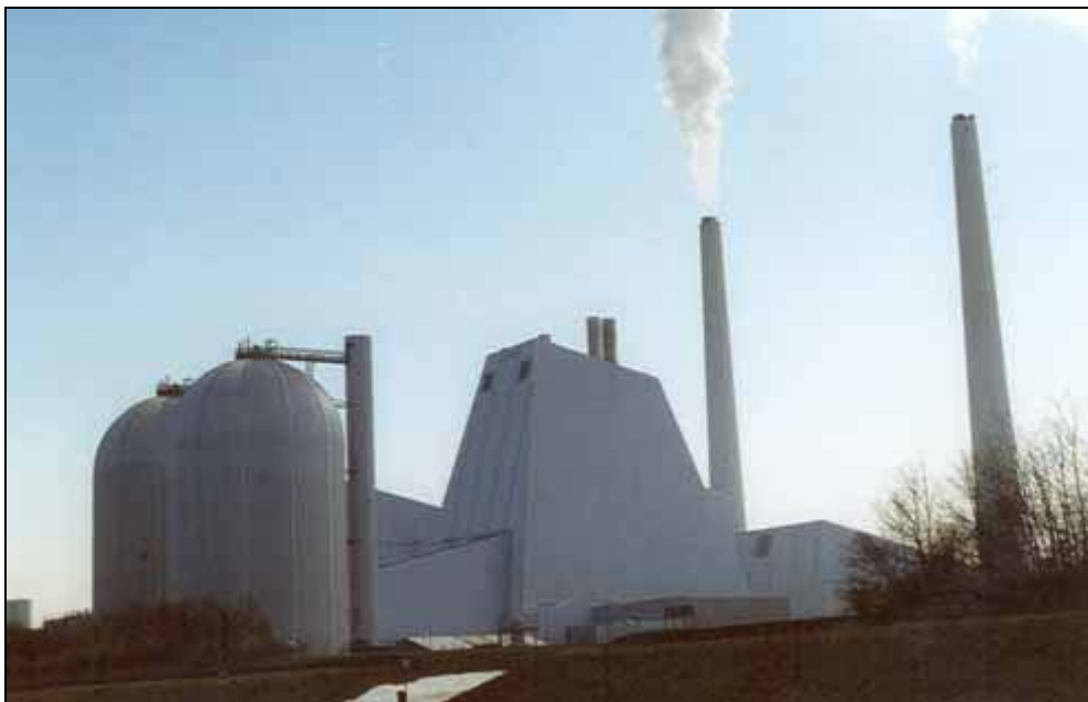
Figure 3.4: Heat storage tanks in connection with a multi-fuel Coal, natural gas, oil, wood chips, straw) 500 MWe cogeneration unit, Avedøre Denmark 21
