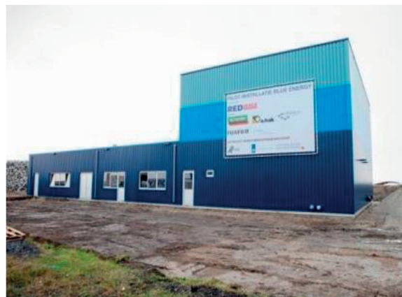
Fig. 34: RED pilot plant at Afsluitdijk, Netherlands. Source: The Daily Fusion 2014
