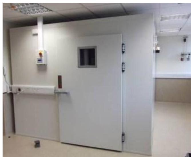
Walk-in freezer chamber in the Hydrates and Ices Laboratory
